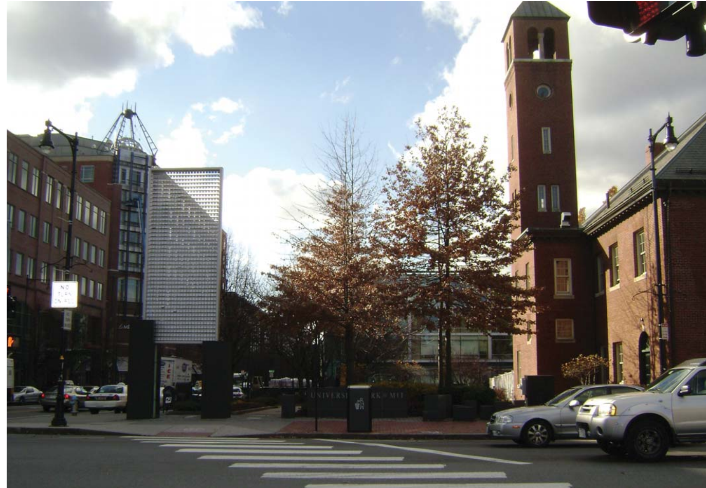
Existing Conditions CORNER OF MASS AVE AND SIDNEY STREET
