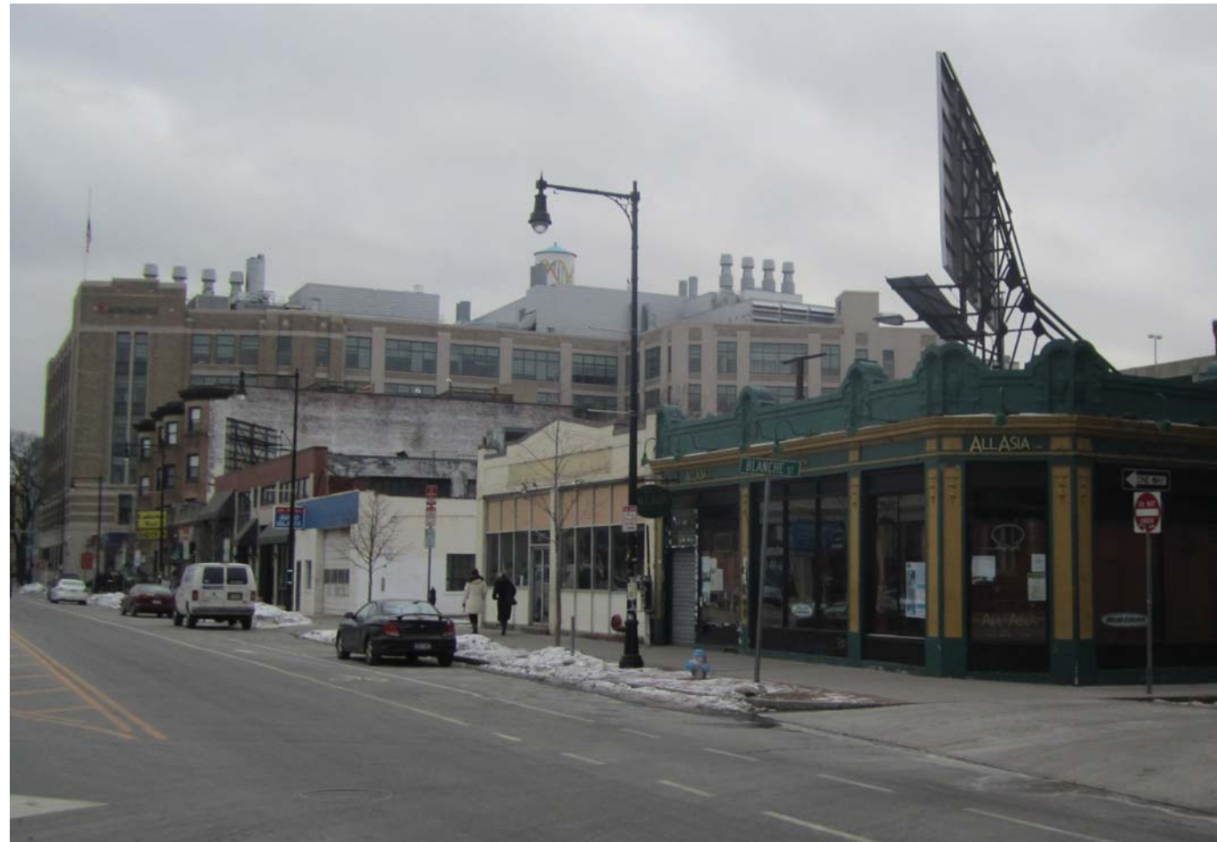
Existing Conditions CORNER OF MASS AVE AND STATE STREET
