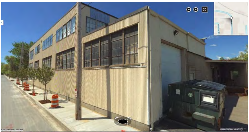
Existing Bldg on 95 Fawcett St.
