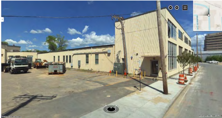
View of site looking North
