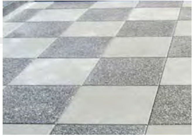
Concrete Pavers on Pedestal System
