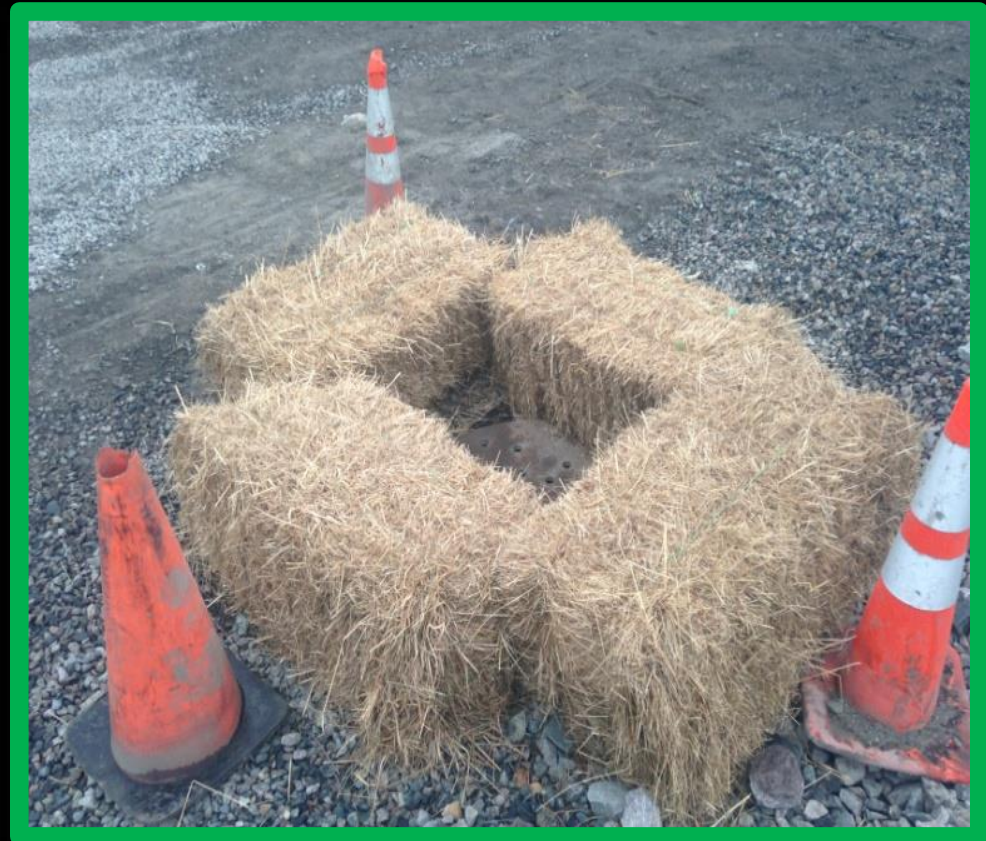
Silt sack with hays
