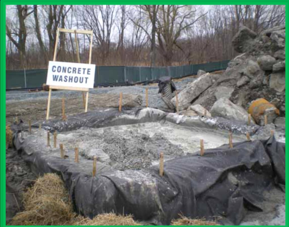
Designated concrete wash out
