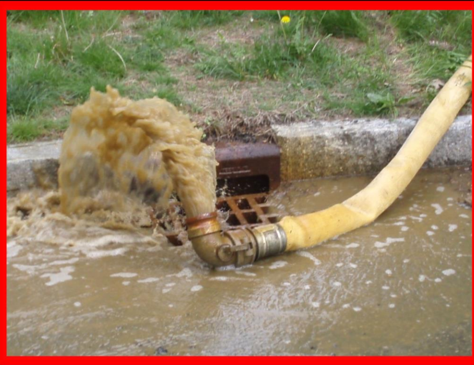
Illegal Dewatering to Catch Basin
