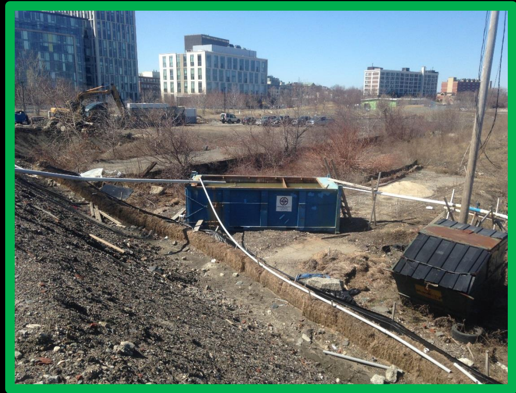
Silt fence/hay bale
