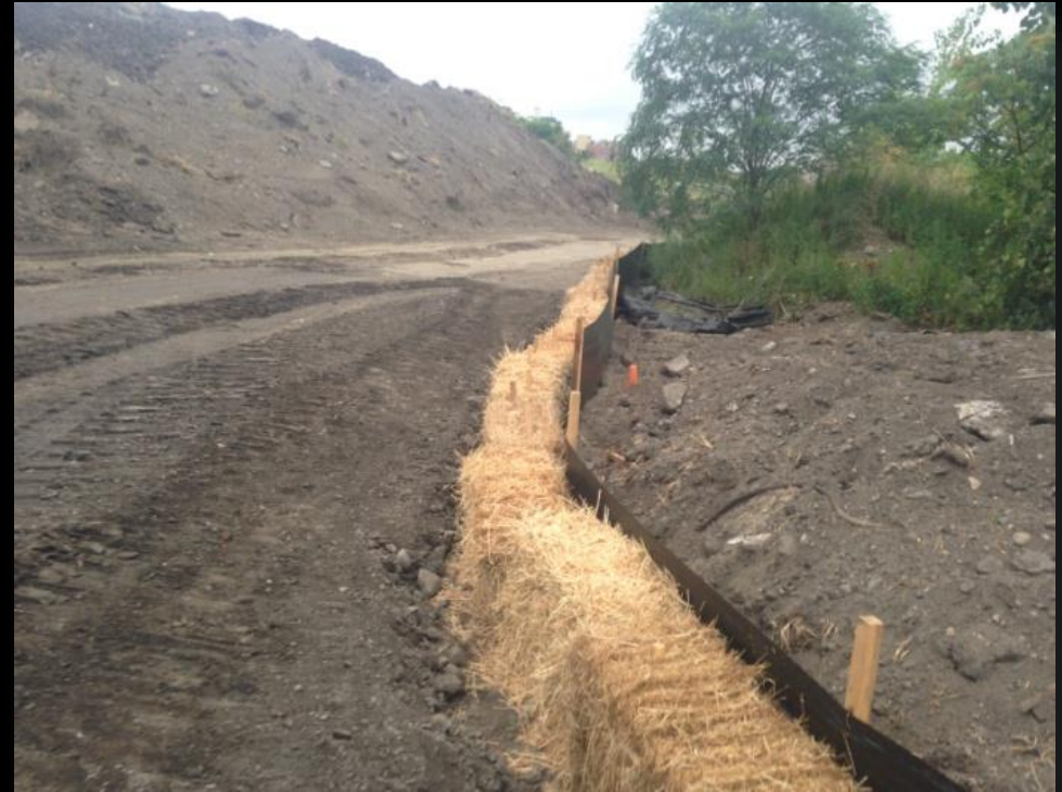
Silt fence/hay bale
