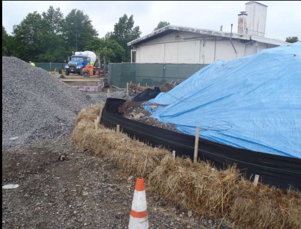
Silt fence/hay bale – staging covered
